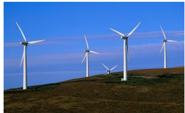
Fig. 4 Wind Turbines in Working.
